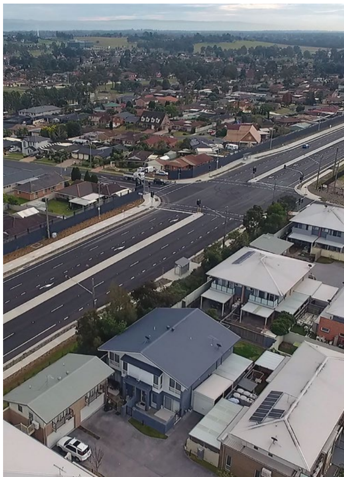
Newly built Werrington Arterial Road
