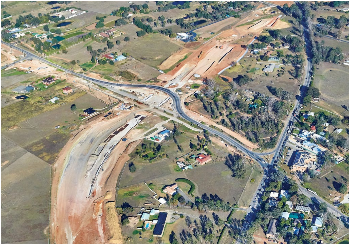
Bringelly interchange looking south
